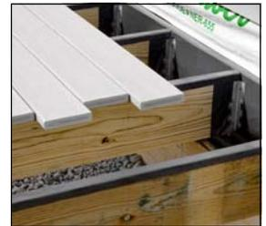
**To protect metal from ACQ-treated lumber:** 3" or 6" DeckWrap is recommended. Apply a protective layer of DeckWrap between the ACQ lumber and the metal. This will prevent the ACQ from corroding the metal. Make certain to use fasteners that are compatible with ACQ lumber.
